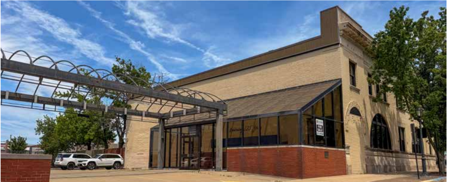
Local developer Corky Joyner has the former Sangamo Club property in downtown Springfield under contract and hopes to convert it into apartments. PHOTO BY ZACH ADAMS
