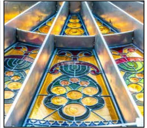
Left: The detail of a quarter section as part of a mockup provided for approval prior to fabricating the stained glass pieces. Center: Steve Brooks produced 300 rondels with variations from light to dark that were used for the inner circle.. Right: The panels laid into the framework. PHOTOS COURTESY B.A. HUDGINS PHOTOGRAPHY
