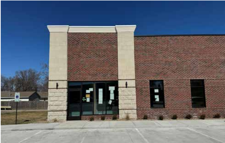
An April opening is planned for an OSF HealthCare clinic in Lincoln, 602 Woodlawn Road. PHOTO COURTESY OF OSF HEALTHCARE
